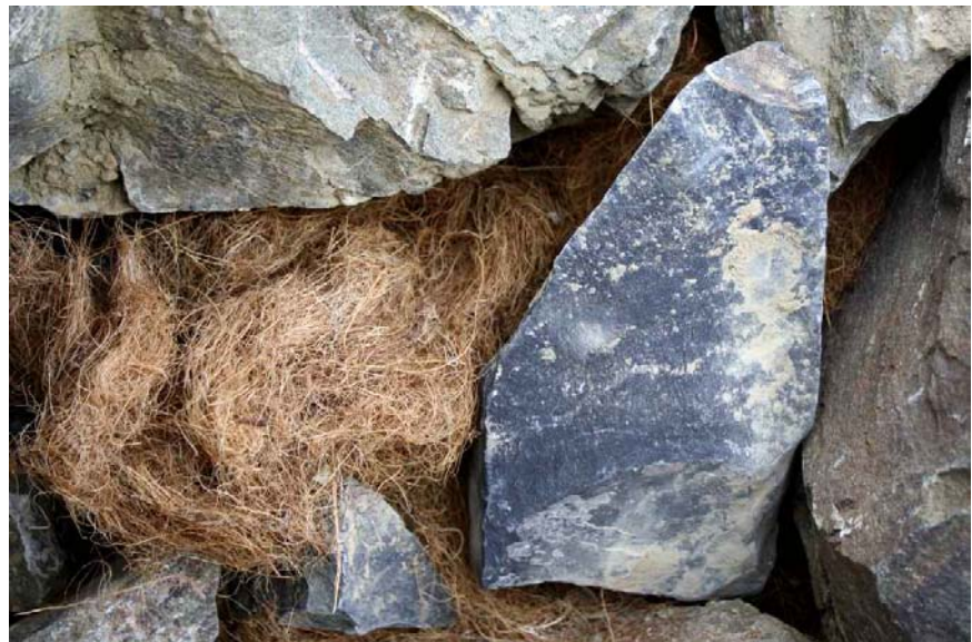
Photo 3. COIR stuffing into larger voids
